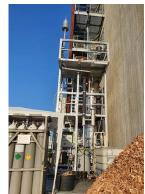
Within the BMWK project "SyntheseReady" the flexibilization of air gasification plants is investigated. To this end, a 100 kW counterflow air gasifier from ReGaWatt GmbH is being modified for oxyfuel operation
